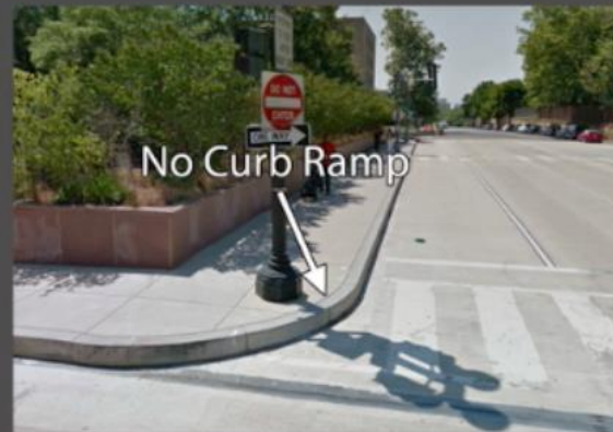
A lack of a curb ramp at this corner obstruct wheelchair users from getting on and off the sidewalk.
