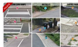
Deep Learning for Sidewalk Assessment 2016 - Present
